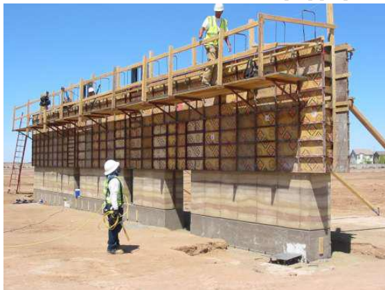
Figure-4: formwork for earth rammed wall [2,1]
